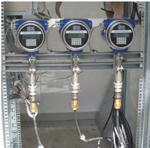
Figure 2-23. Cable gland example with braided shielded cable
