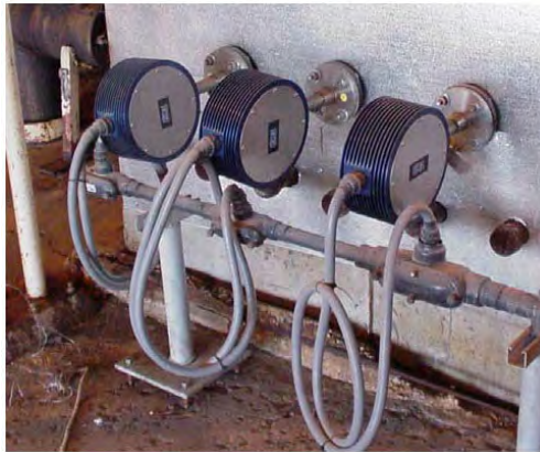
Figure 2-21. Flex sensor connection for service loop, TA version using liquid tight conduit
