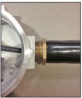
Figure 17: Torquing the Cable Gland
