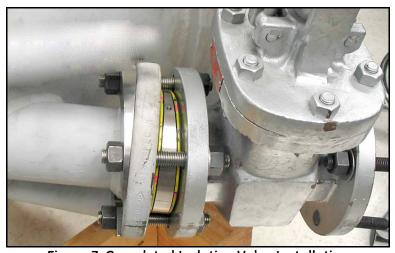
Figure 7: Completed Isolation Valve Installation
