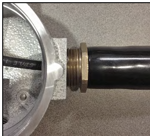
Figure 9: Torquing the Cable Gland
